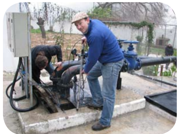
Installation of monitoring system at the Hazzir spring, Salt, Jordan (Foto: N. Goldscheider, KIT)
