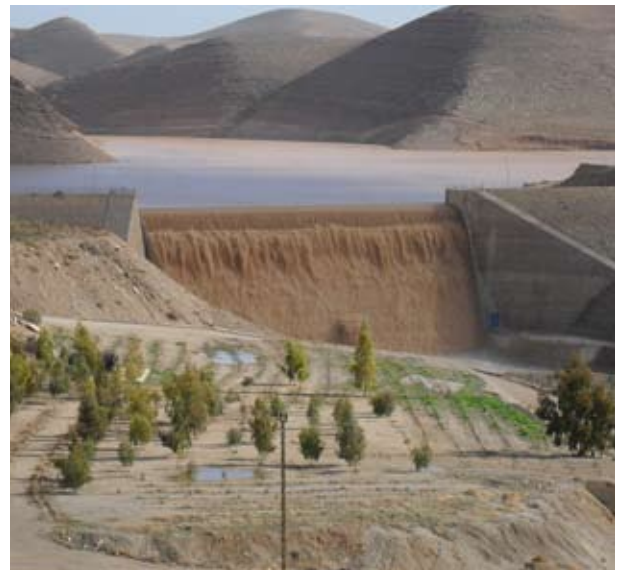
Wadi Wala (Jordan) with dam and reservoir for flood water storage (Foto: A. Sawarieh, KIT)
