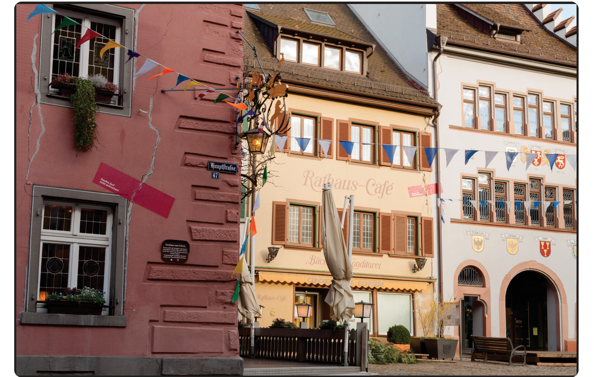
Staufen im Breisgrau, damaged houses as a result of ground heave after thermal drillings.
