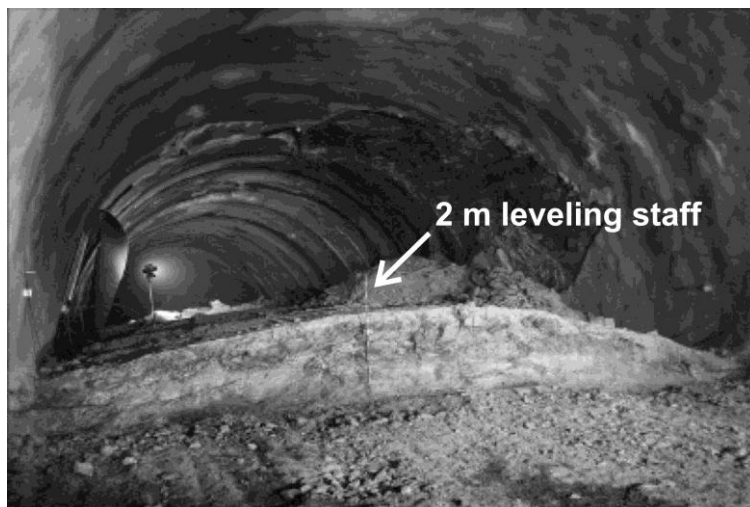
Figure 1: Floor heave in the Chienberg road tunnel during construction. During an interruption of the excavation works, the floor of the top heading experienced a heave of about 1.5 m within three months. Photo courtesy of Aegerter & Bosshardt AG, Basel.
